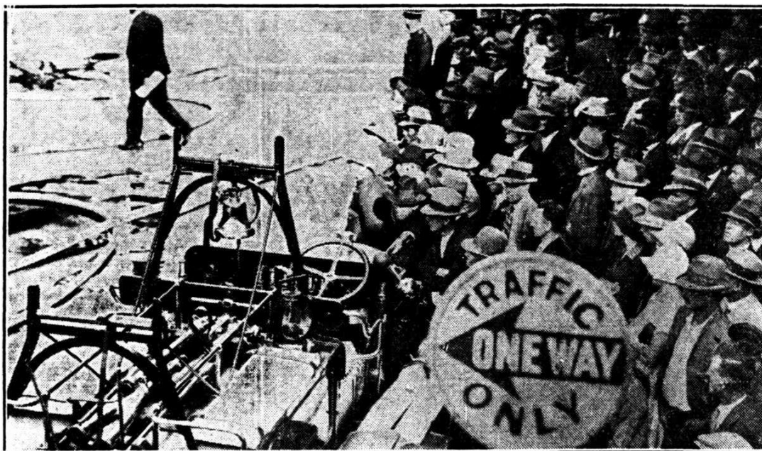
SPECTATORS WATCH FIREMEN COMBAT BLAZE IN HINDLEY STREET TODAY When a fire broke out in Adelaide House this morning a large number of people gathered. Policemen kept everyone at a safe distance. In the left foreground is one of the appliances brought to the scene by members of Metropolitan Fire Brigade.
